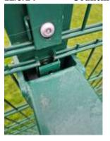
...." the tightening of the mesh retaining nuts.
